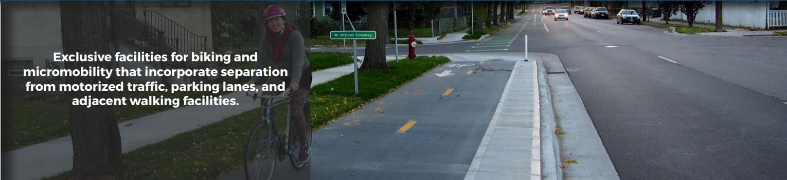
**Exclusive facilities for biking and micromobility that incorporate separation from motorized traffic, parking lanes, and adjacent walking facilities.**
