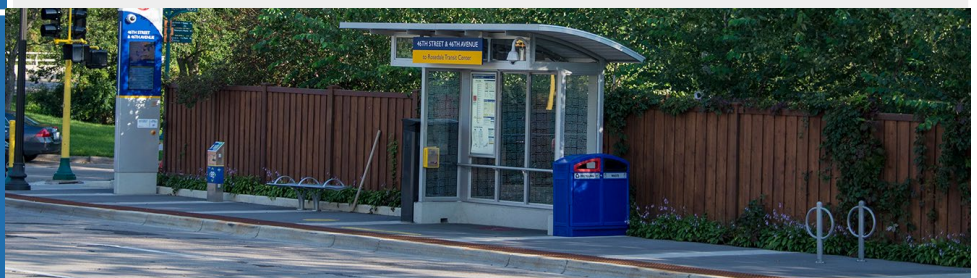
Figure 3.5C.2: Constrained situation BRT station with smaller shelter and combined boarding area and pedestrian clear zone
