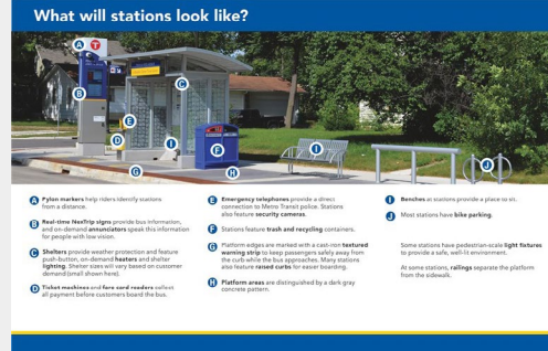
Figure 3.5C.1: Elements of Bus Rapid Transit stop
